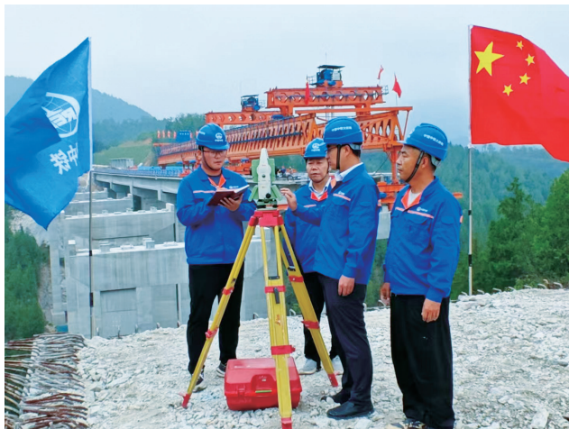
● 监测桥梁线形
